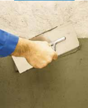
Application with trowel
