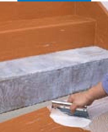
Applying Ultrabond Aqua-Contact on the back of PVC flooring
