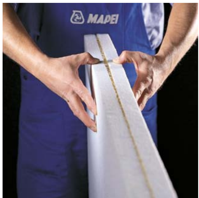
Bonding polystyrene foam panels
