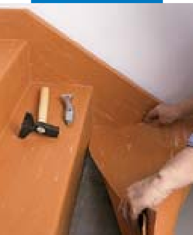
Laying PVC flooring
