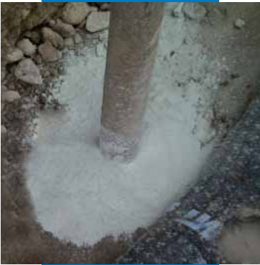
Application of Mapeproof Seal around through piping
