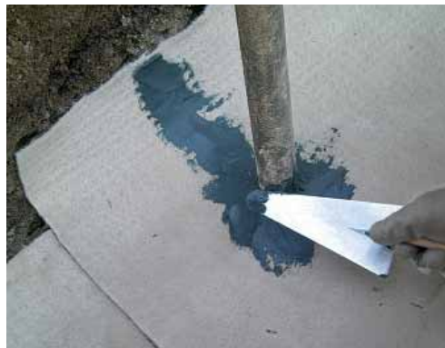
Fig. 1 - Application by trowel of Mapeproof Mastic around through piping
