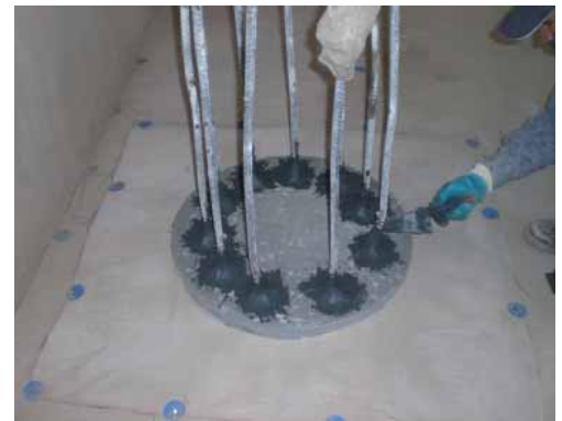
Fig. 2 - Application of Mapeproof Mastic around reinforcement rods in pile heads
