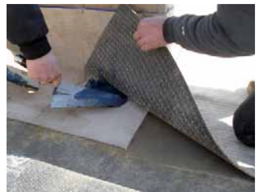
Fig. 6 - Sealing between Mapeproof bentonite sheets with Mapeproof Mastic
