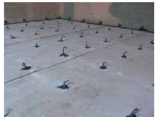
Fig. 4 - Grouting connection rods with Mapeproof Mastic
