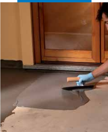
Waterproofing of terraces by trowel
