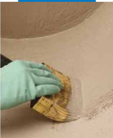
Waterproofing of terraces by brush
