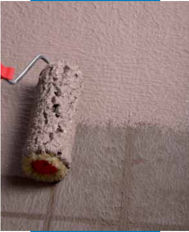
Waterproofing of terraces by roller
