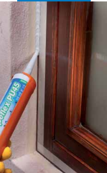
Flexible sealing of joints
