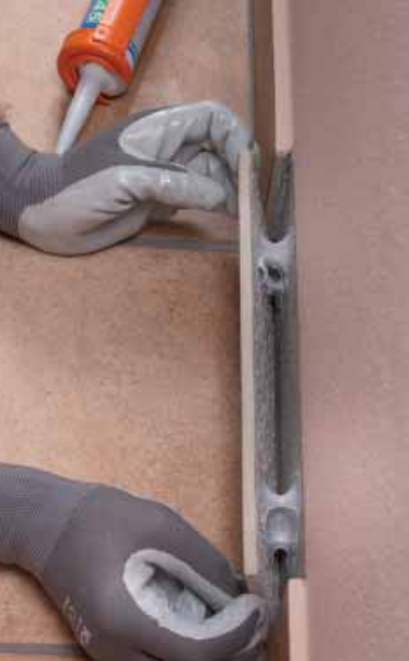
Flexible bonding of elements
